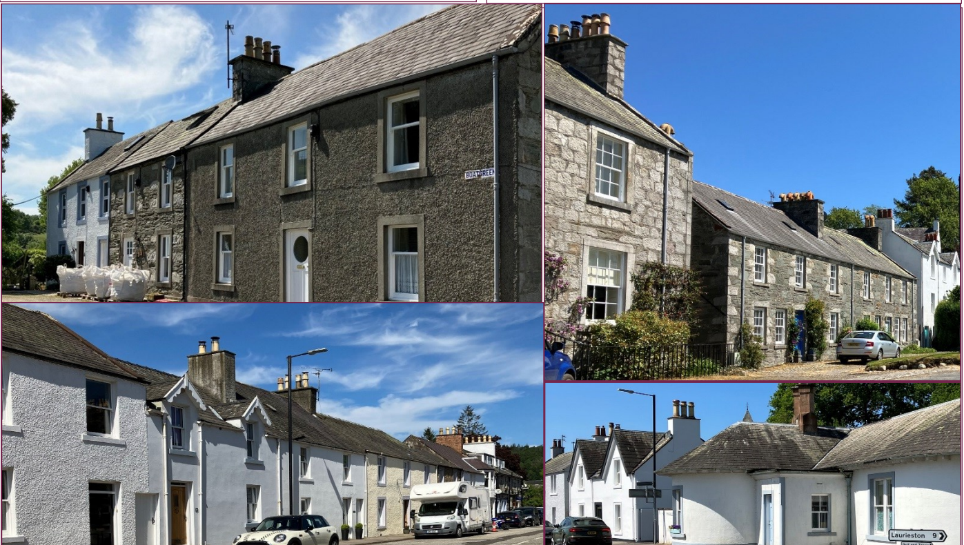
Clockwise from top left: A selection of elevations of buildings from Boatgreen, Ann Street, Woodside Terrace and the western end of Fleet Street.
