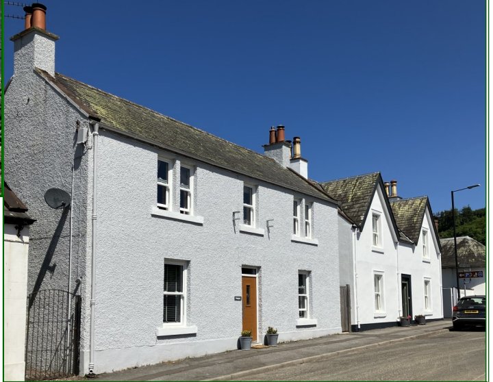
Above: B Listed Angel Hotel from the late 18 th century; Classical proportions and features painted whinstone elevations with painted sandstone window margins and quoins and a painted stone string course.
